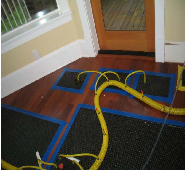
DURING Combination of 8 Point (which were modified by cutting between the grid sections) & Multi-Port Panels
